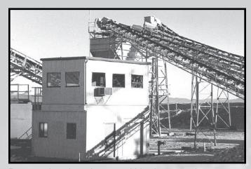
Personnel and equipment within the control rooms are isolated from high termperatures, dirt and noise. The building is self-contained, complete with emergency power systems, housing the computerized operating system at this automated cement batch plant.
