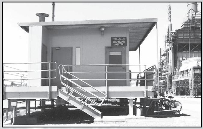
Elevated to eliminate hazards from heavier-than-air gases, the **Permit Series** Functional Building is located at the refinery production process. It contains a quality control chemical laboratory, lavatory and kitchen area. Air conditioning is provided through a pressurized system which simultaneously filters hazardous chemical vapors and purges the interior space.
